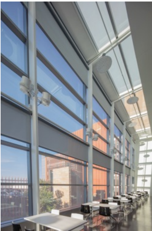
TZ100 Zipper Tension System skylight installed at the Stephen M. Ross School of Business at the University of Michigan. (Photo Credit: Bob Perzel)
